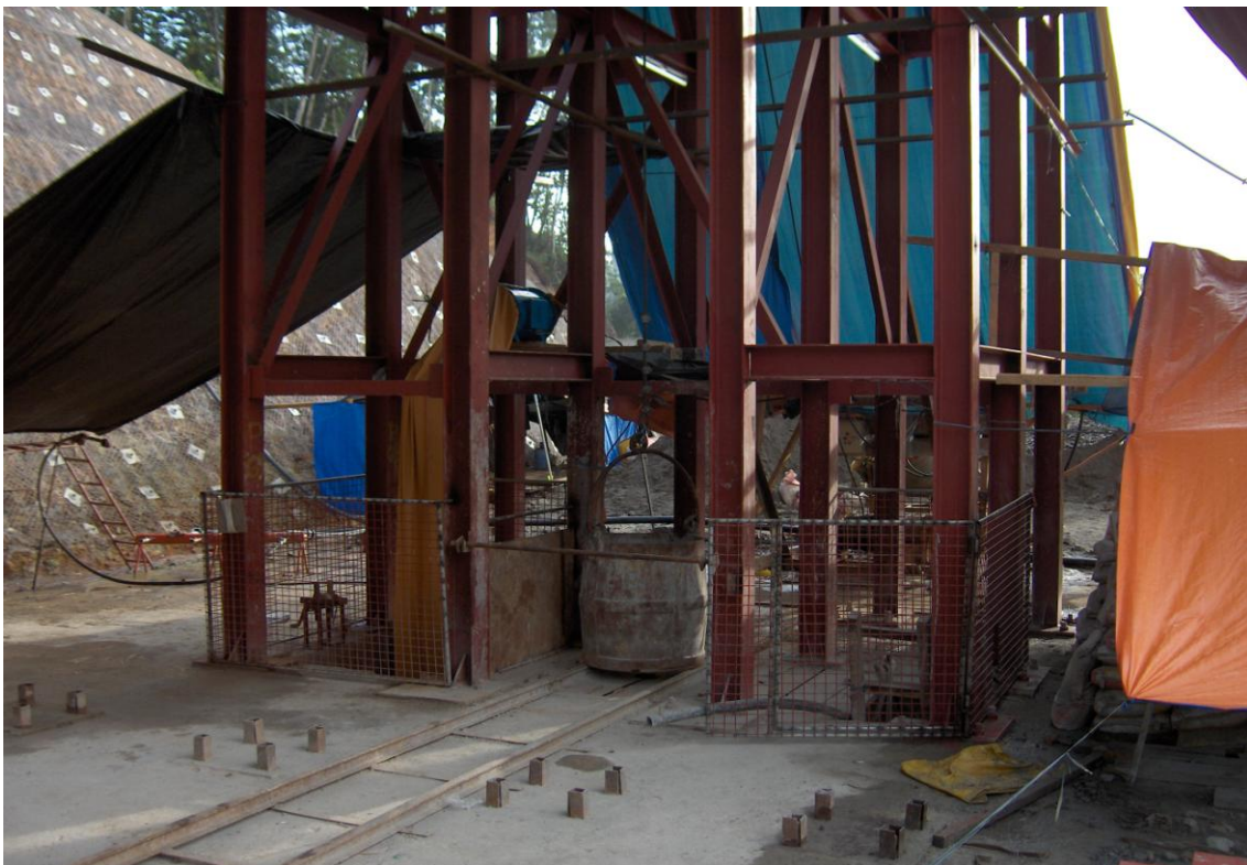
Plate1. Saga Shaft collar area and temporary headframe
