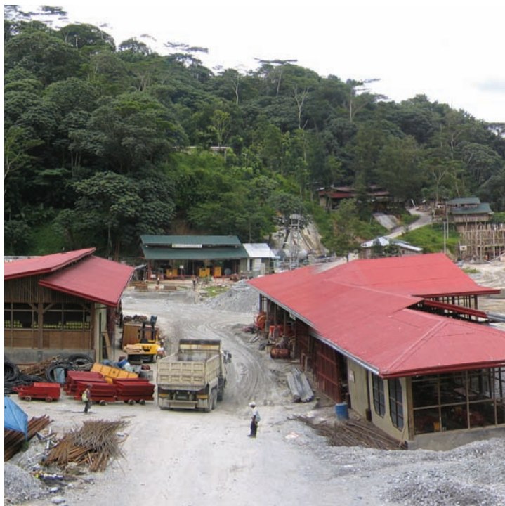
Co-O mine infrastructure
