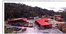
Co-O mine infrastructure
