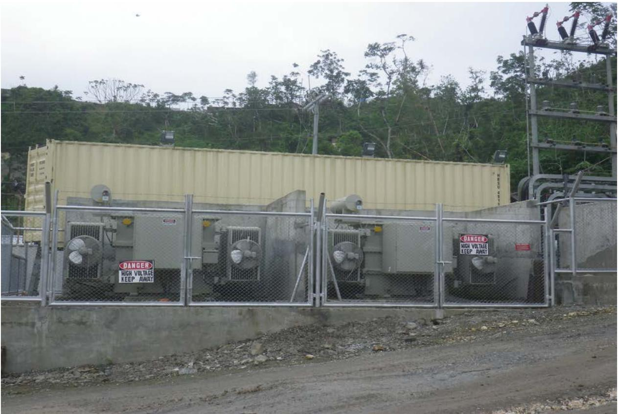
Photo 5. Mine transformer station.
