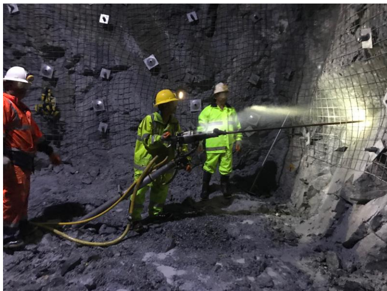
Photo of miners bolting walls of final blast
