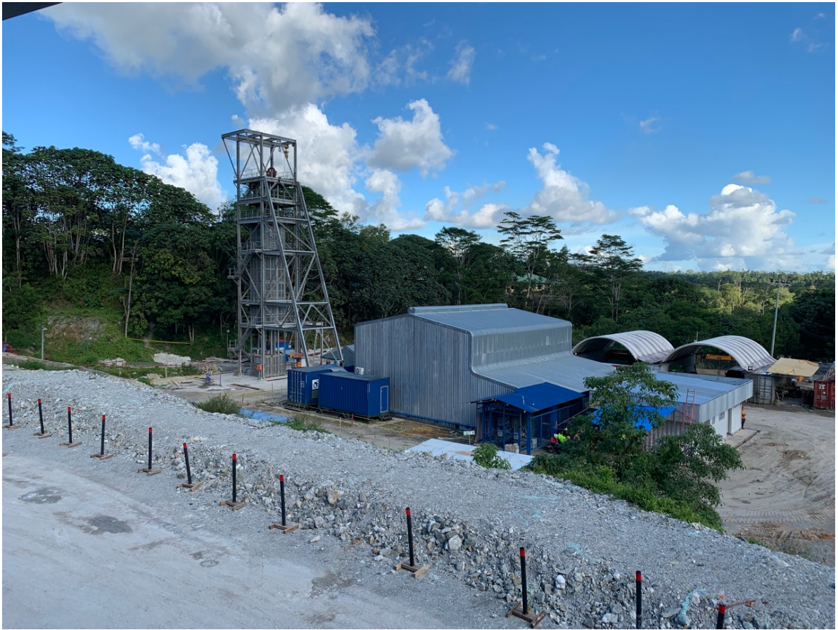
Figure 1: Completed E15 Service Shaft and surface infrastructure
